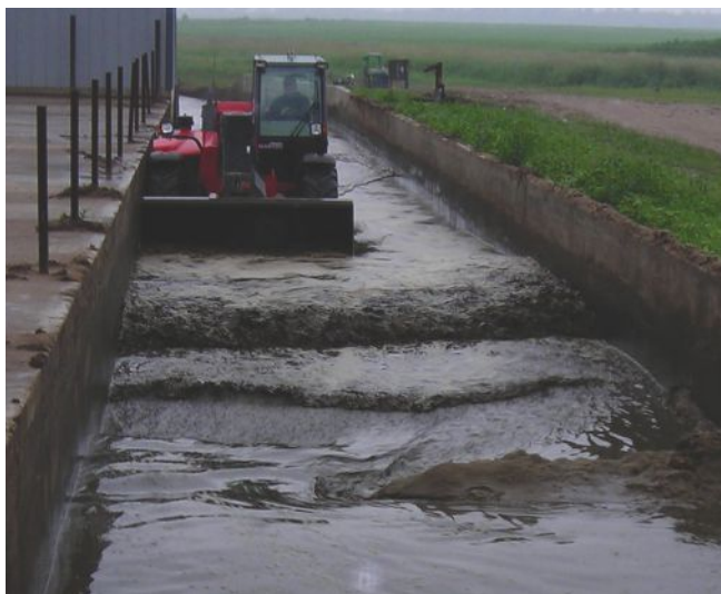
Payloader working in a conventional sand settling lane.
